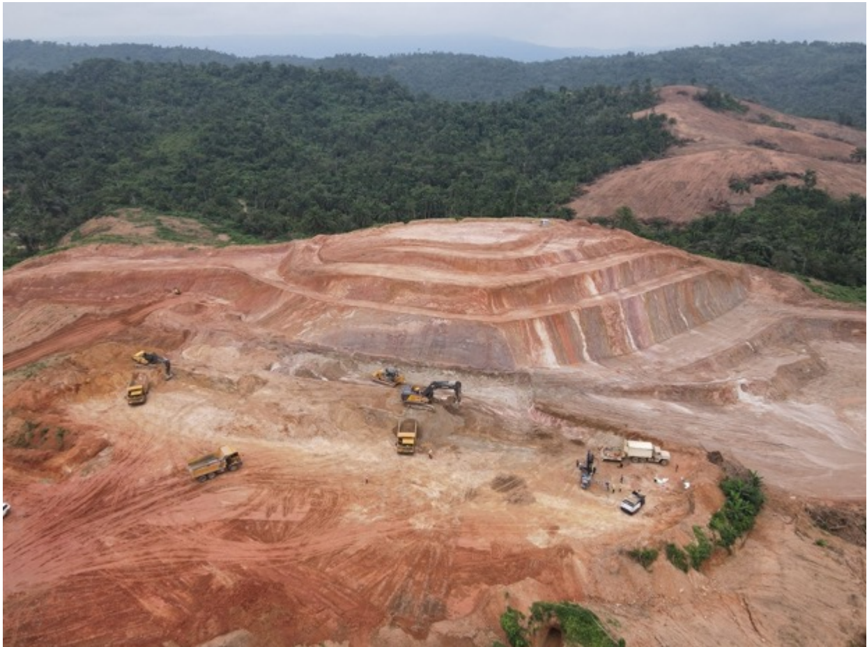
Figure 4: Segilola Pit Excavation
