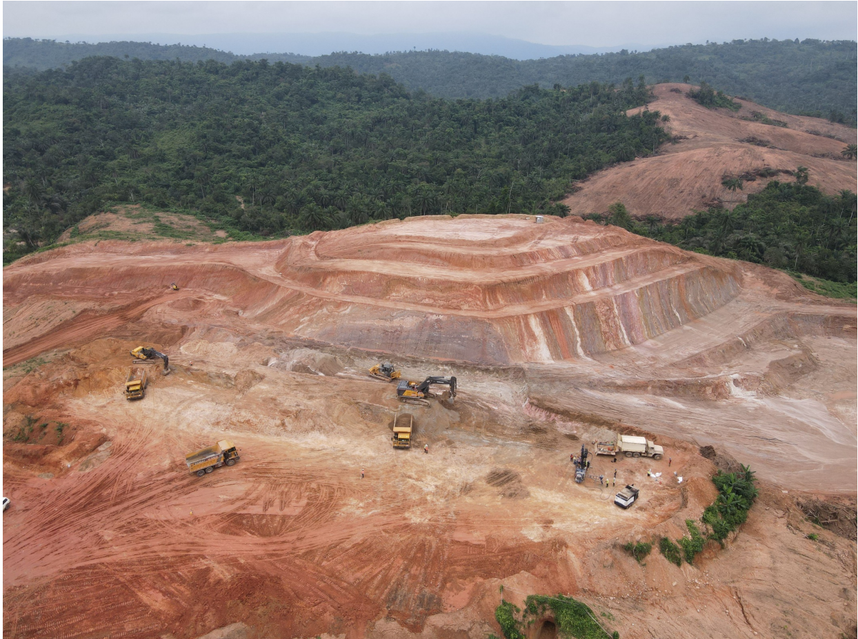
Figure 4: Segilola Pit Excavation
