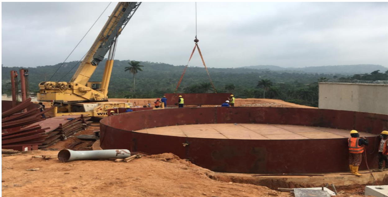
Figure 1: Installation of the Reclaim Water Pond
