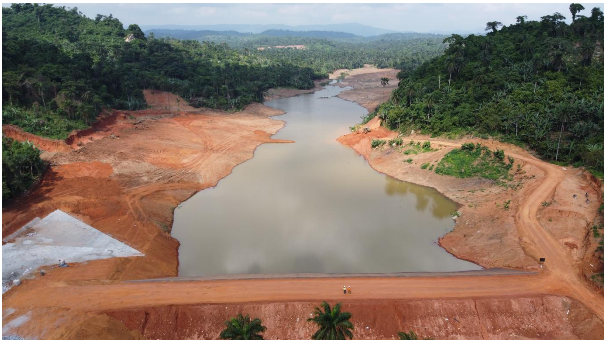
Figure 3: Water Storage Dam and Water Storage Facility
