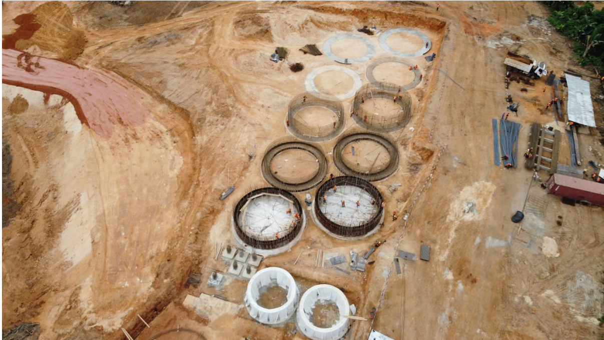
Figure 2: Leach tank construction progress
